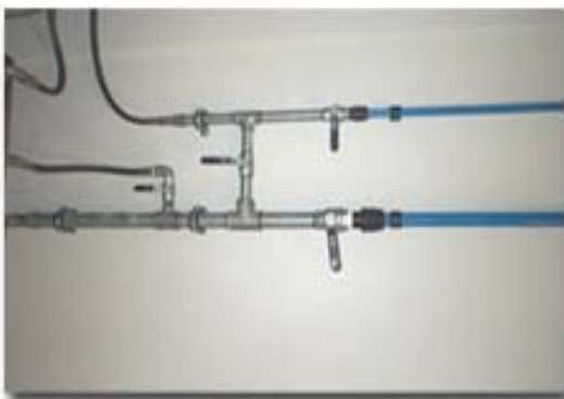
Equal elbows example of use : obstacles bypass... and offset drops
