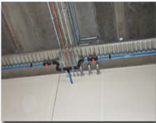
Equal elbows example of use : obstacles bypass... and offset drops
