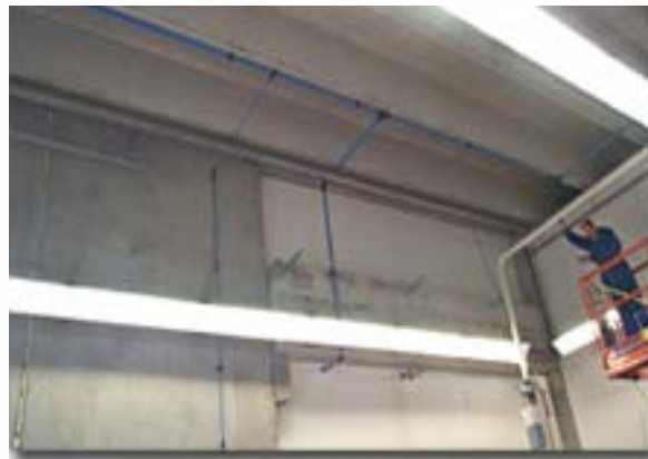
Equal elbows example of use : obstacles bypass... and offset drops
